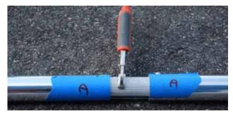
**STEP 4** - Squeeze the sleeve with vice grips and slide the two pipes over the slotted sleeve until they touch the vice grips.
